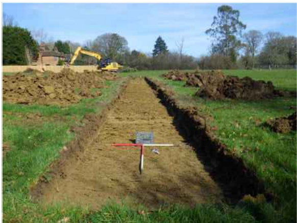
Trench 19 facing north east
