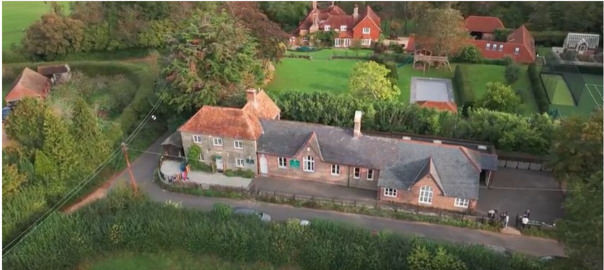
Ashurst C of E Primary School: elevated view from the south
