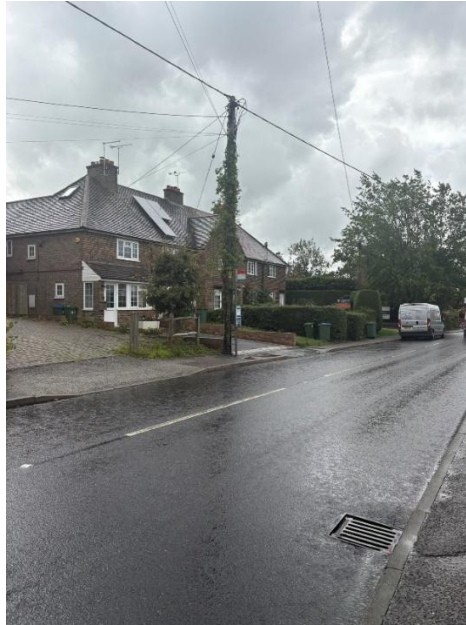
Photograph 1: Existing Conditions Along Henfield Road (Looking South-East)
