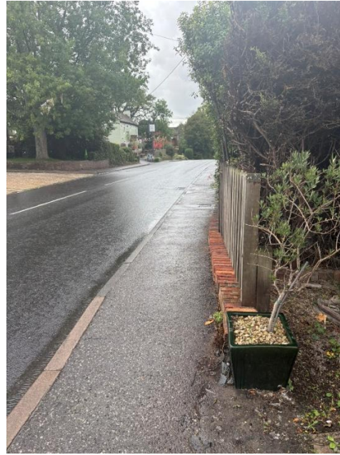
Photograph 4: Pinch Point Along the Footway
