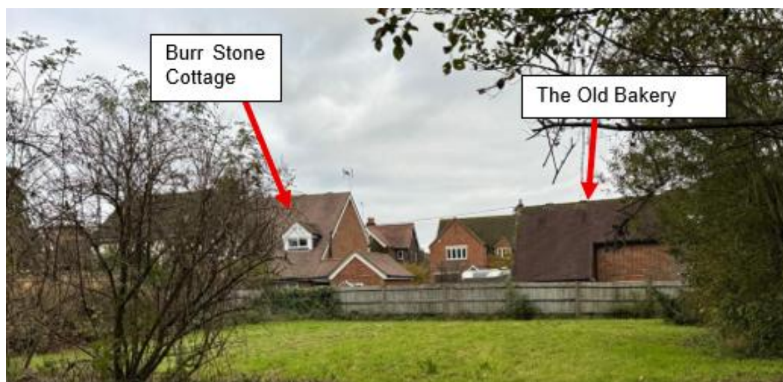
Figure 11 - Photograph of Dwellings to the East
