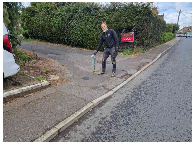
Location of pipe 21.5m US of CP6, depth 1.49m
