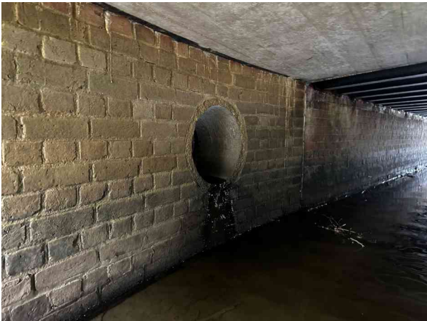
Outfall to stream
