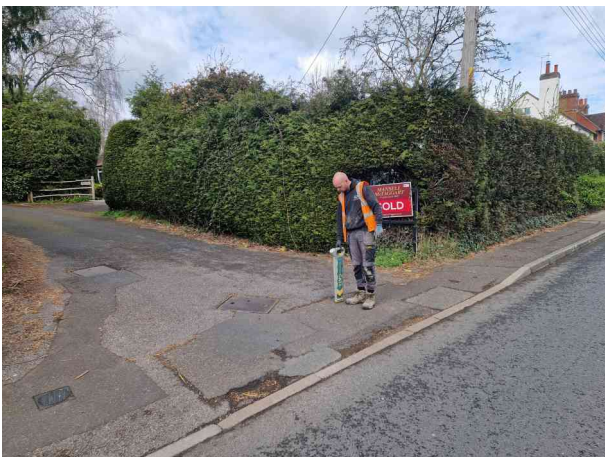
Location of pipe 23.7m US of CP6, depth 1.29m
