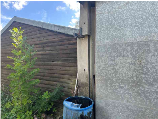
Open gutter to butt
