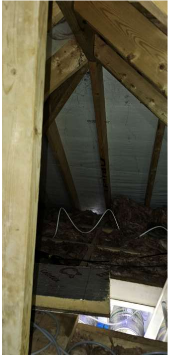
Loft hatch above ground floor beer 'cellar'
