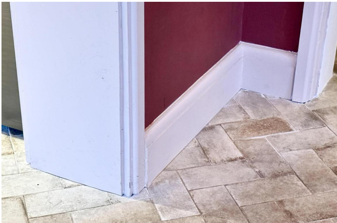
Fig 4: The large nibs at the side of the wall still allow for the division of this space to be understood, in the context of the historic floorplan of the dwelling. Skirting and architraves have been replicated to match.
