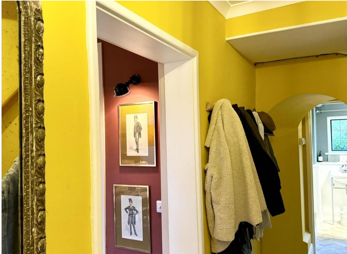
Fig 5: The original doorway leading from the hallway into the kitchen has been boarded over as a stud wall, sitting behind the coats on the wall. This is considered to be a reversible intervention.
