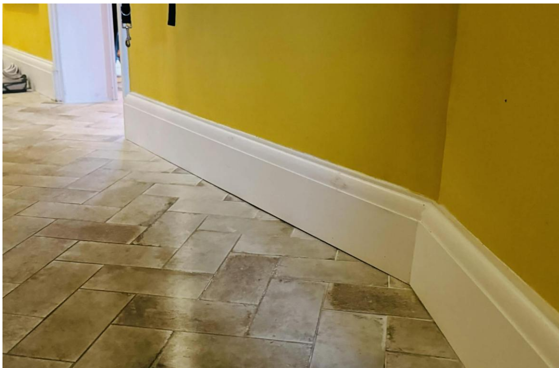
Fig 6: The infill of the former doorway has been achieved seamlessly and with a matching skirting board. This change is a reversible intervention in accordance with Historic England guidance.
