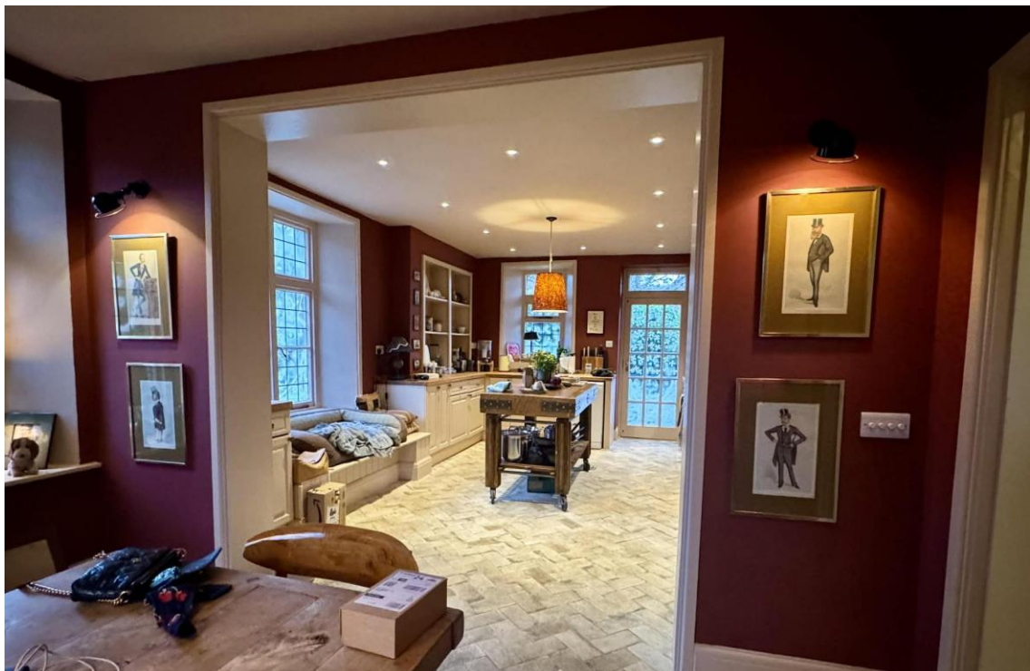
Fig 2: The view from the dining room looking into the kitchen. As a retrospective application, the former partition wall has been opened up, leaving large nibs and a ceiling beam to distinguish between the two.
