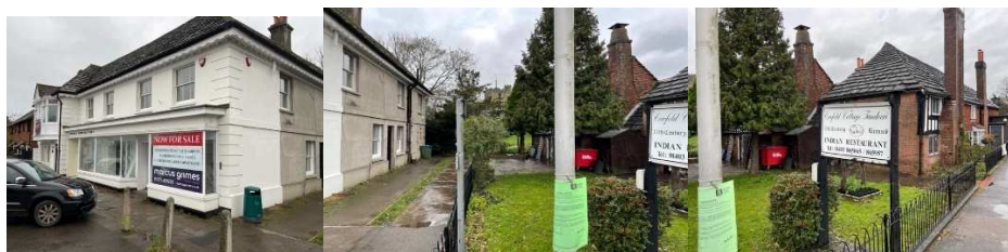
Frontage – Cowfold Stores, Passage to St Peter’s Church, St Peter’s Cottage
