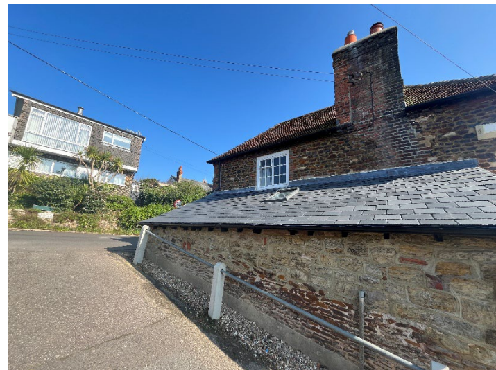
Plate 13: Single-storey extension on west side of the cottage.
