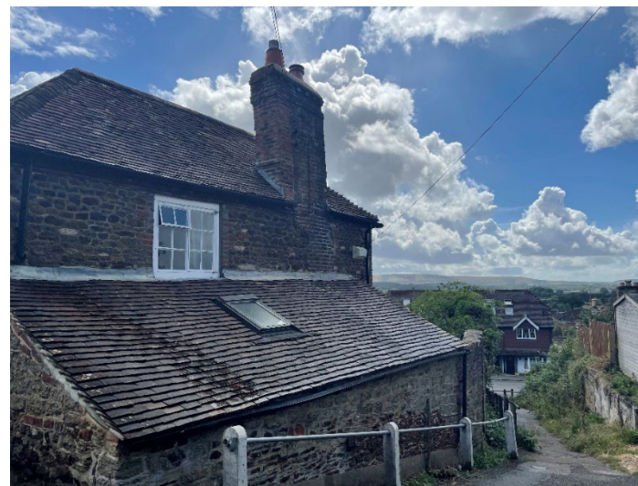
Plate 24: North-westerly extension prior to the works.
