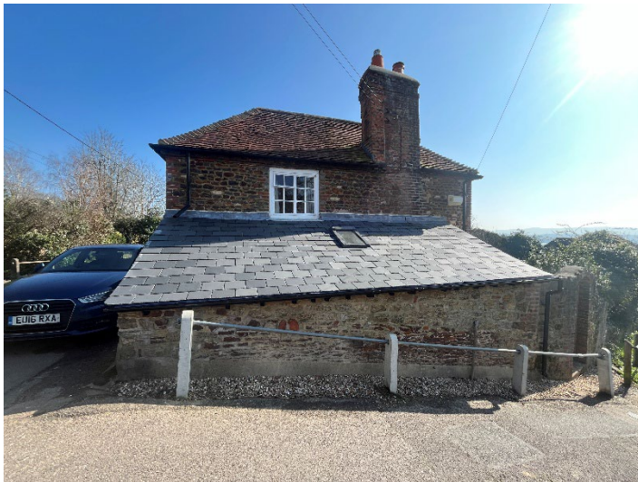
Plate 26: The re-roofed north-westerly extension, 2026.
