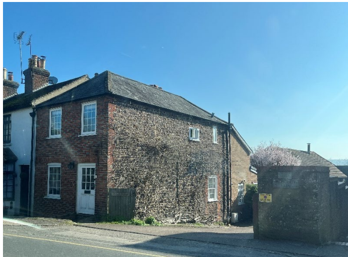
Plate 23: Rubble stone, red brick and slate roofs.
