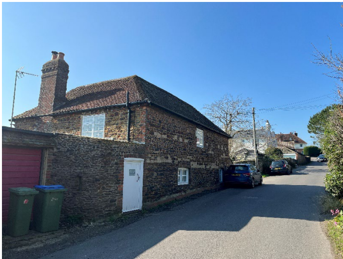
Plate 11: Single-storey extension to east side of cottage left of frame.
