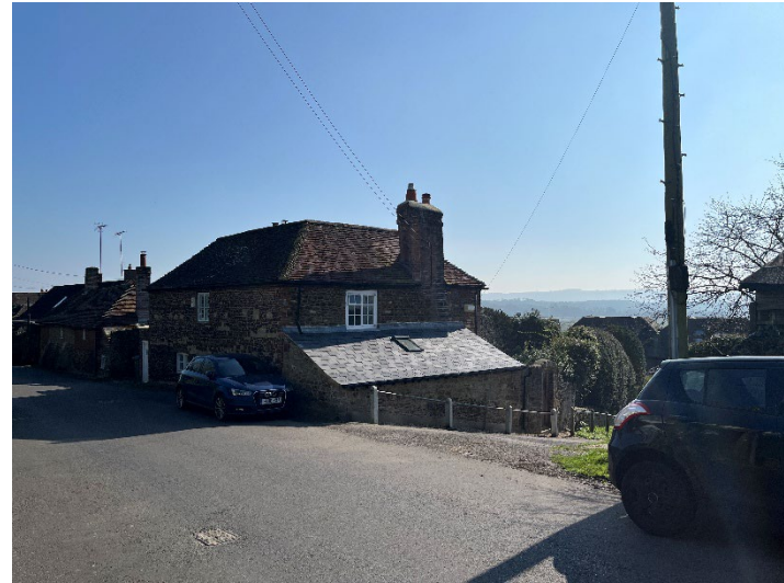
Plate 12: Single-storey lean to extension on west side of the cottage.
