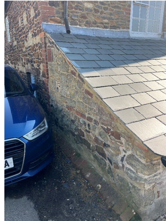
Plate 27: Verge detailing of the re-roofed extension, 2026.
