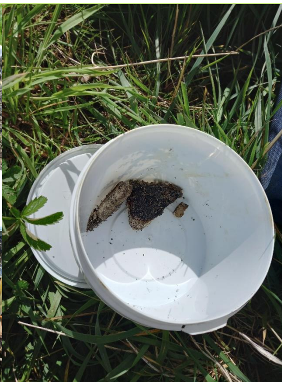
Photo 10: HP3 possible ACM (AIB?)
