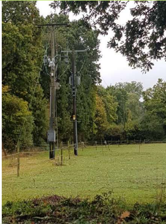
Photo 16: Overhead cables in southern field along eastern boundary
