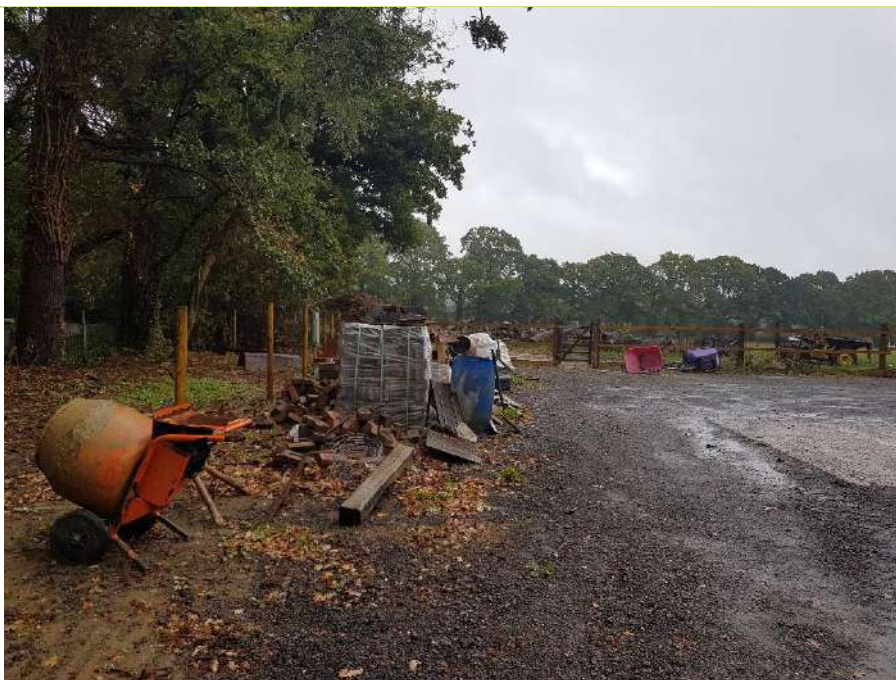
Photo 2: Road subbase hard standing, for drive around to stables. Northern field of site in distance. (stables out of shot to the left)
