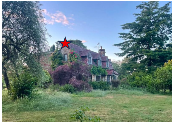
Photograph 13 – View at the start of the second survey on 2 nd June 2026 for surveyor three by the corner on the front southeast elevation and side northeast elevation. Red star – indicates location of the common pipistrelle emergence.
