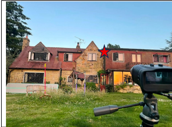
Photograph 19 – View at the start of the third survey on 24 th June 2026 for surveyor three by the corner on the front southeast elevation and side northeast elevation. Red star – indicates location of the common pipistrelle emergence. Red star – indicates the location of two common pipistrelle emergences.
