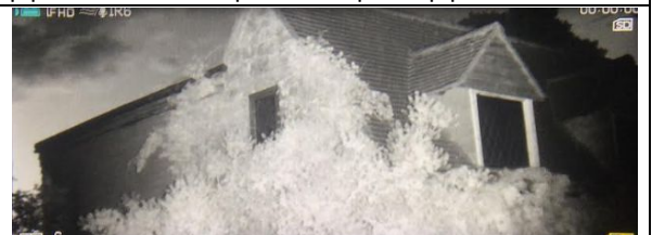
Photograph 6 – View at the start of the first survey on 11 th May 2026 for surveyor three by the corner on the front southeast elevation and side northeast elevation.
