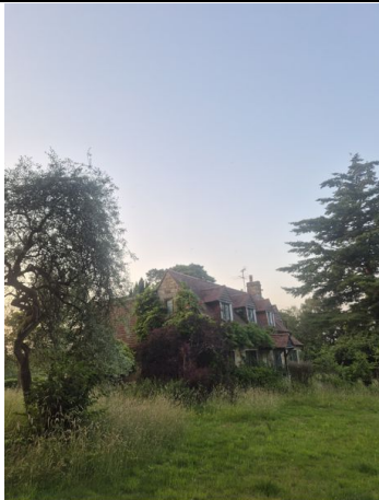
Photograph 15 – Camera view at the start of the third survey on 24 th June 2026 for surveyor one by the corner on the front southeast elevation and side southwest elevation.
