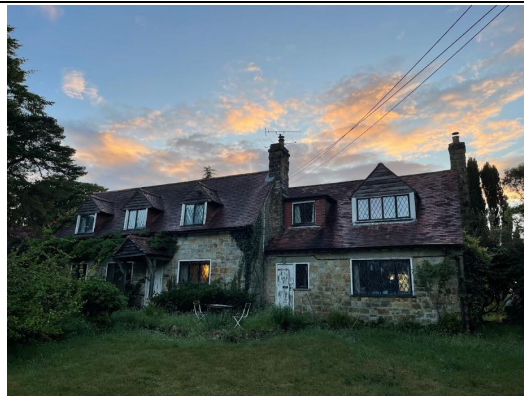
Photograph 11 – View at the start of the second survey on 2 nd June 2026 for surveyor two by the corner on the front southeast elevation and side southwest elevation.
