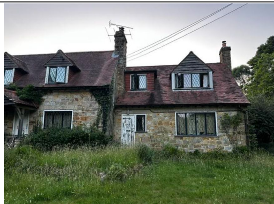
Photograph 17 – View at the start of the third survey on 24 th June 2026 for surveyor two by the corner on the front southeast elevation and side southwest elevation.
