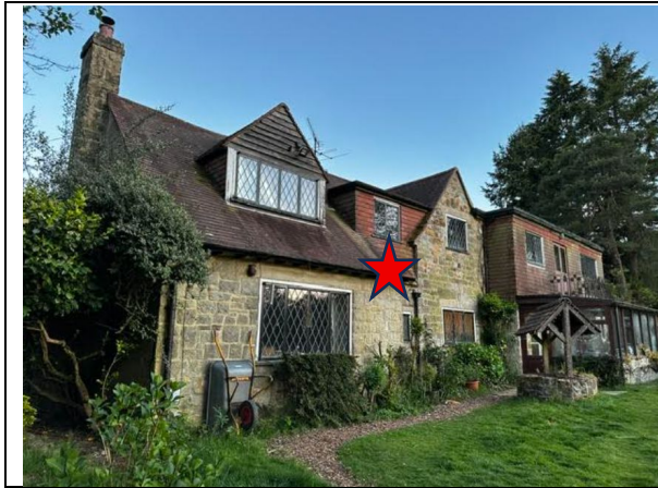
Photograph 1 – View at the start of the first survey on 11 th May 2026 for surveyor one by the corner of the rear northwest elevation and side southwest elevation. Red star – indicates possible pipistrelle emergence.
