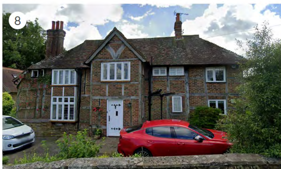
Vicarage Cottage - Grade II Listed
