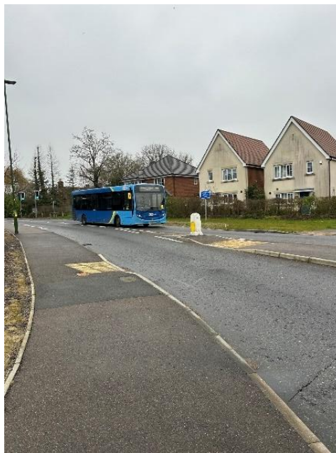
Photograph 3: Pedestrian Crossing on Mill Straight
