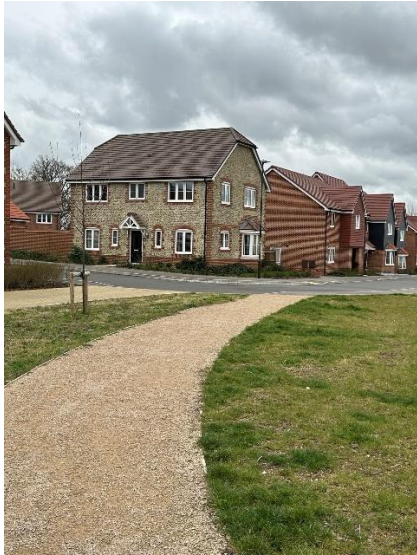
Photograph 7: Footway in Mulberry Fields Development
