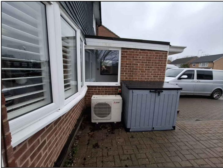
5 - Porch side view
