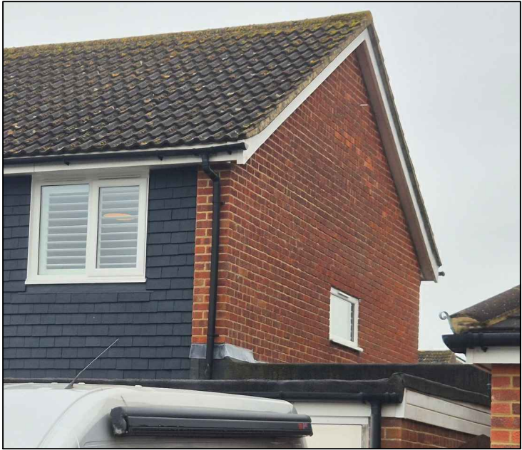
6 - Window on side view
