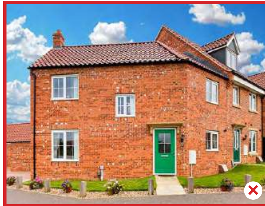
Lack of variation combined with poor roofline continuity
