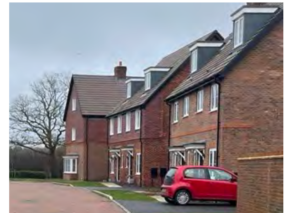
Dormer windows and chimneys add interest to the roofscape
