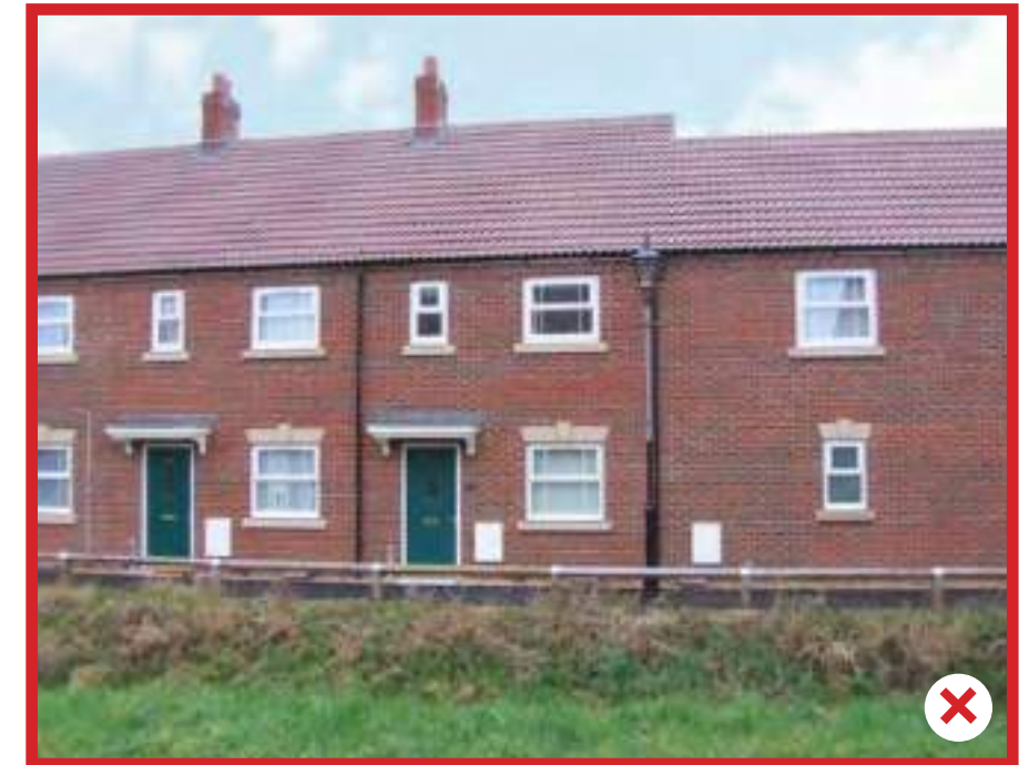
Inconsistent alignment and rhythm along terrace and group rooflines
