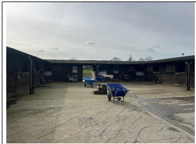
Photograph 3 – Concrete courtyard between the stables.
