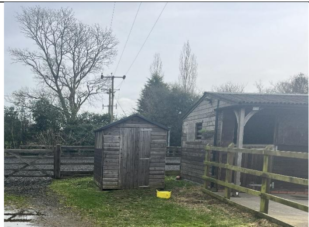
Photograph 13: Exterior of timber shed.
