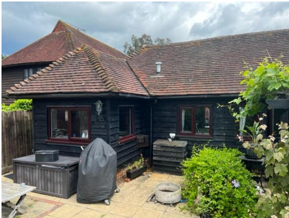
Figure 3. Existing end element, showing the tiled roof and weatherboarded walling.
