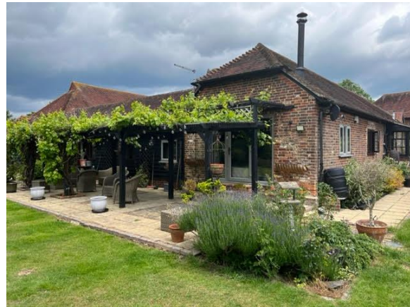
Figure 4. Brick cross-wing and pergola viewed from the private garden.
