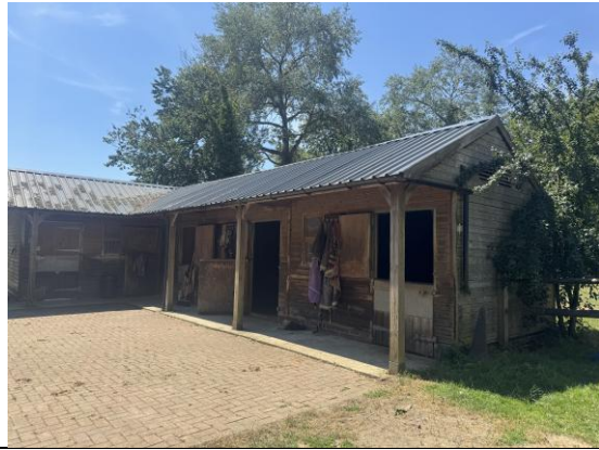
Stables (B1) to be demolished.
