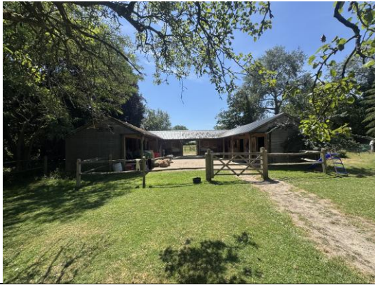
Stables (B1) to be demolished.
