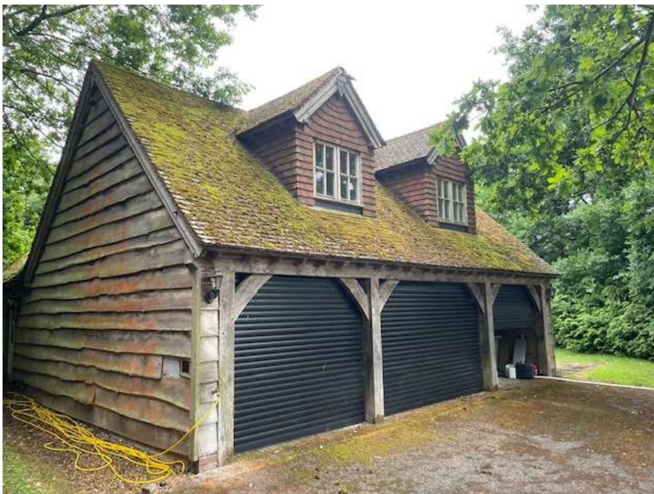
Front elevation of existing building – proposed single storey extension set back from façade on right edge of this photo up against conifer.
