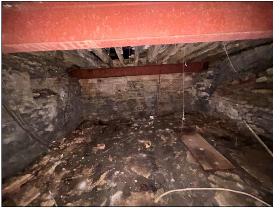
Photo 9: Basement area below the shop floor looking towards the front of the shop
