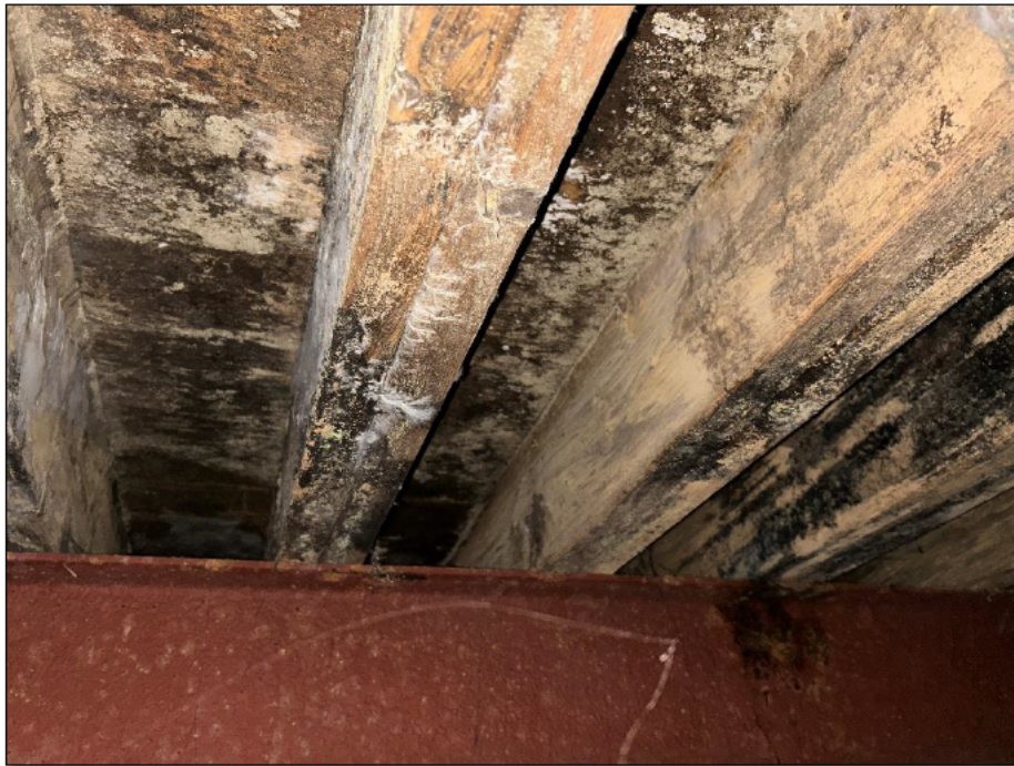
Photo 13: Existing floor joists over basement.
