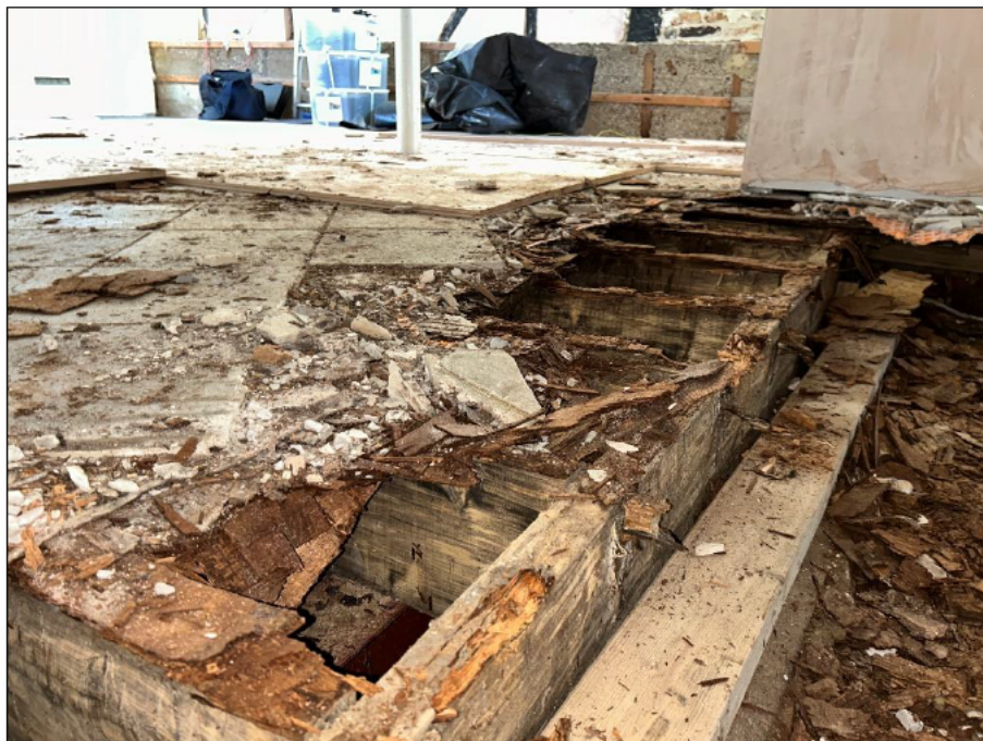
Photo 8: Exposed section of suspended timber floor
