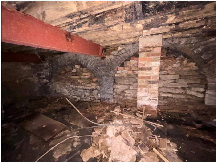
Photo 11: Blocked up arches to vaults.
