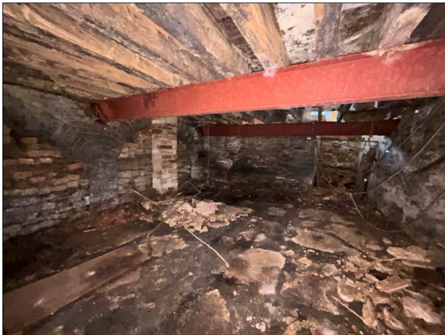
Photo 10: Basement area looking towards the back of the shop
