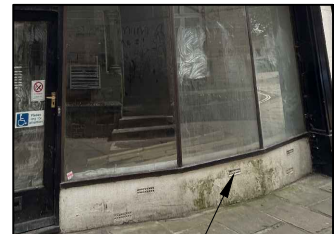
Shopfront: existing airbricks to remain
