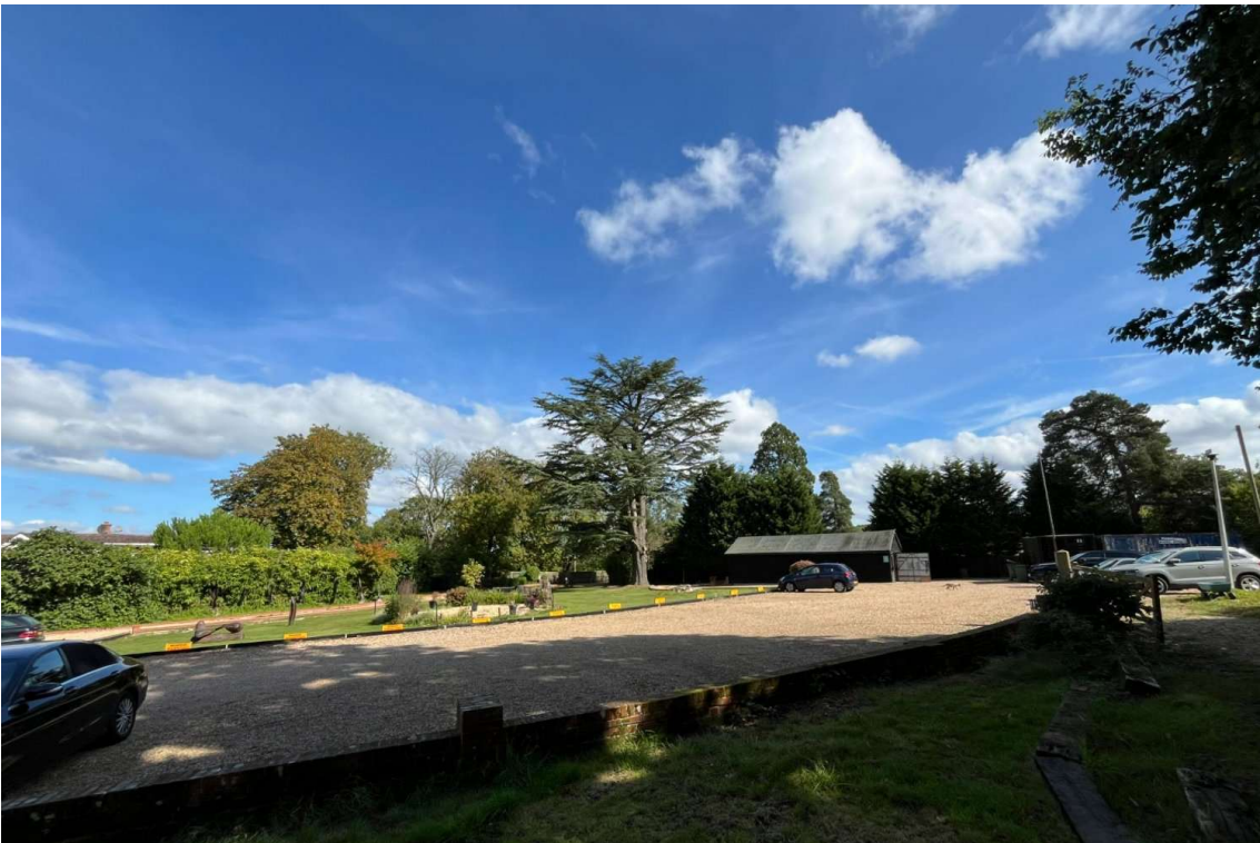
FIGURE 3 - VIEW TOWARDS OUTBUILDING/ STORAGE SHED
