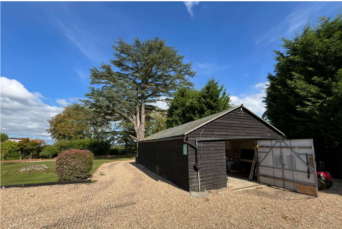
FIGURE 5 - OUTBUILDING/ STORAGE SHED
