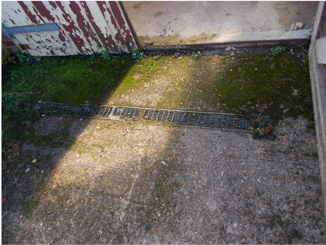
Strip drain in front of garage
