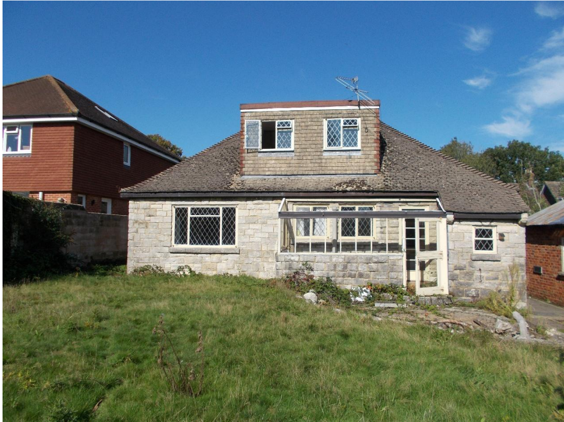
Rear of bungalow
