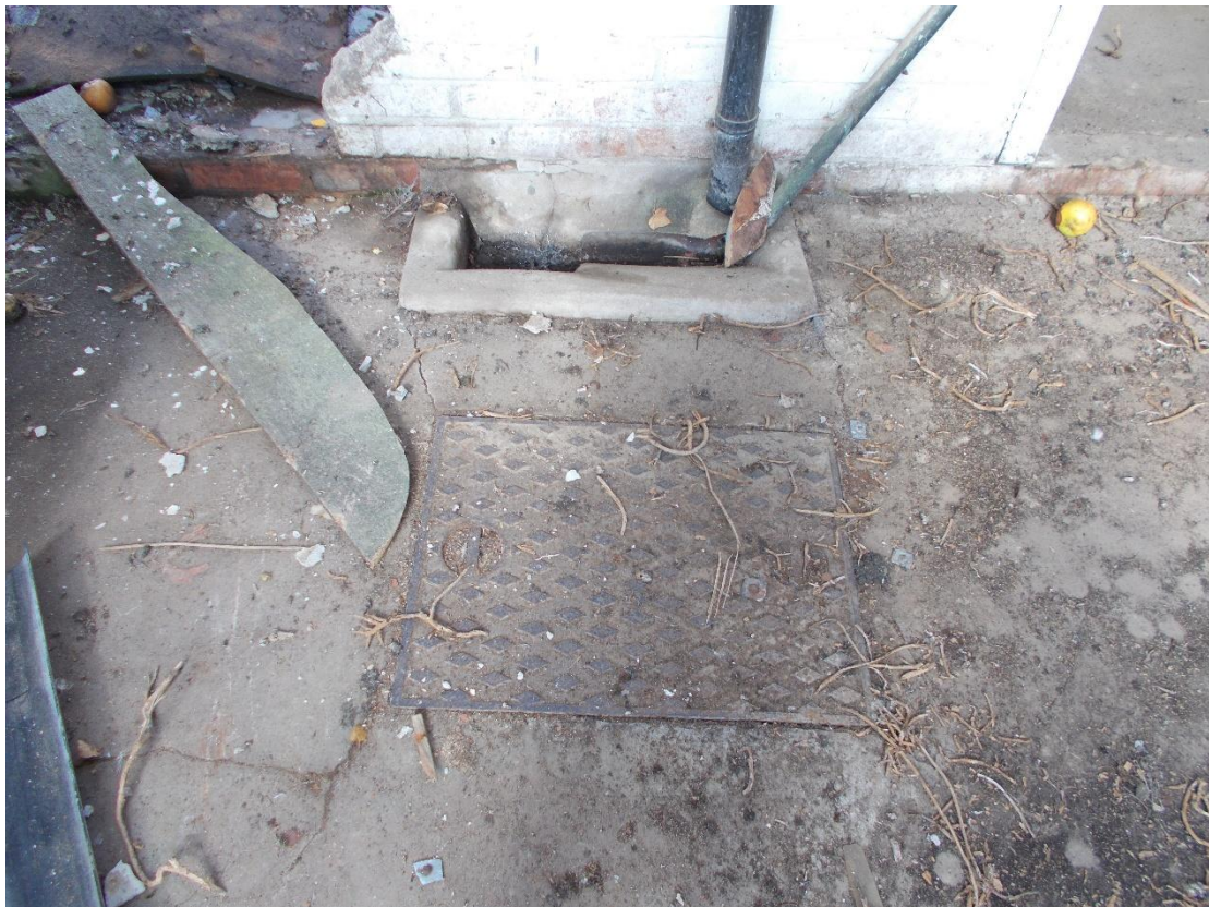
Drainpipe downpipes in garage
