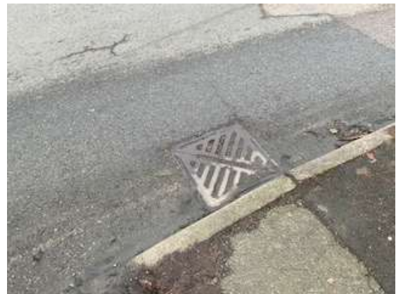
Figure 3: Blocked gully to the northeast of the crossing point.
