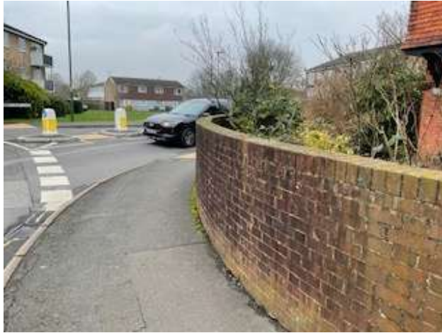
Figure 4: Wall restricting intervisibility at proposed crossing point.
