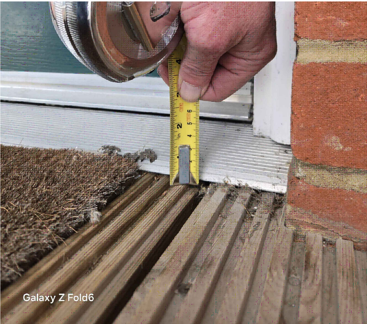
Current door had a ramped threshold, any step will be reduced by the thicker decking
