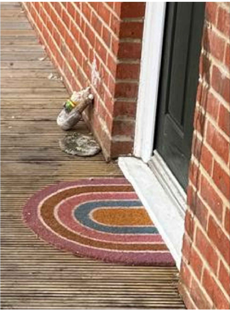
Current door had a step, this will be reduced by the thicker decking
