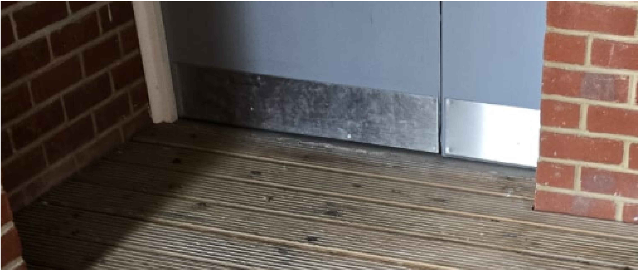
Current door had a step, this will be reduced by the thicker decking
