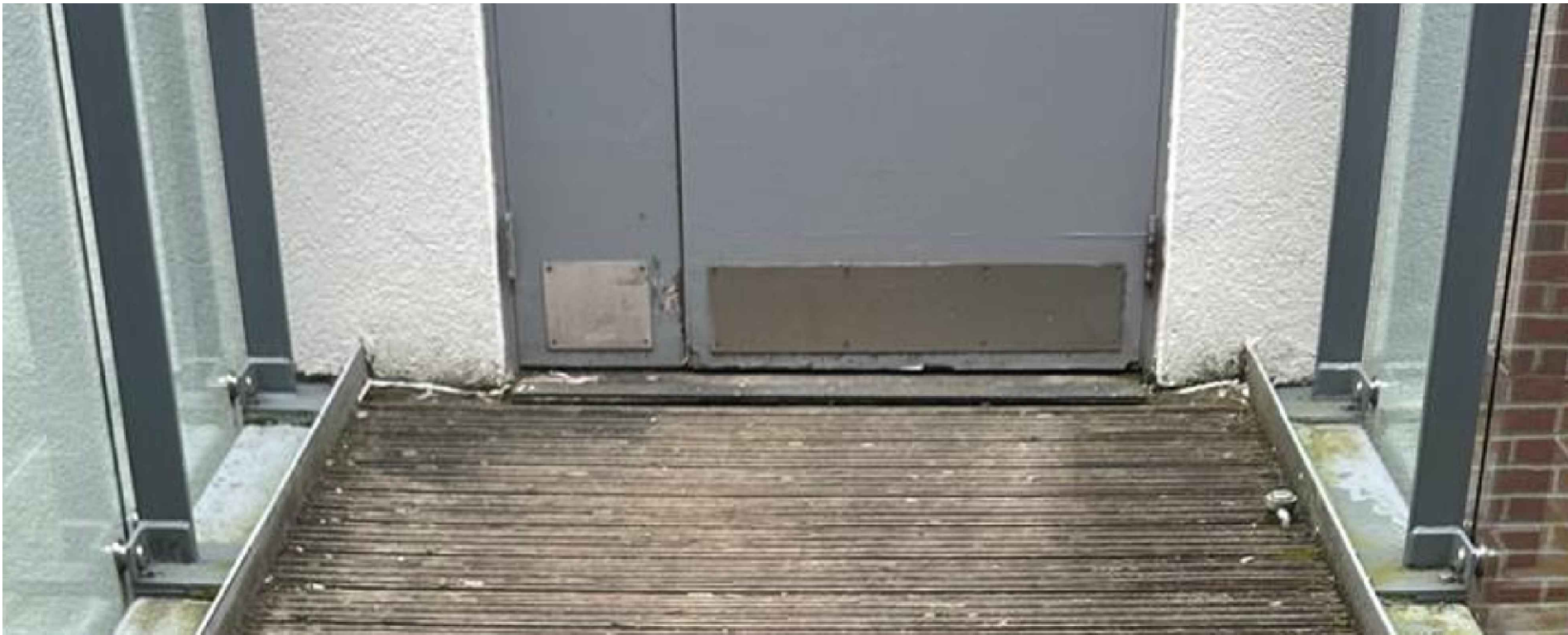
Current door had a step, this will be reduced by the thicker decking
