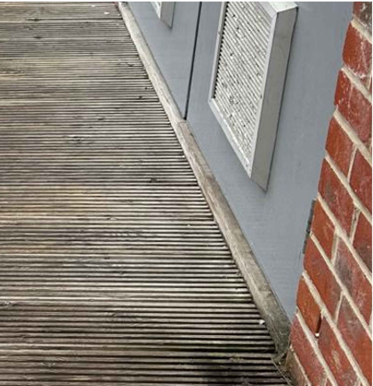
Current door had a step, this will be reduced by the thicker decking
