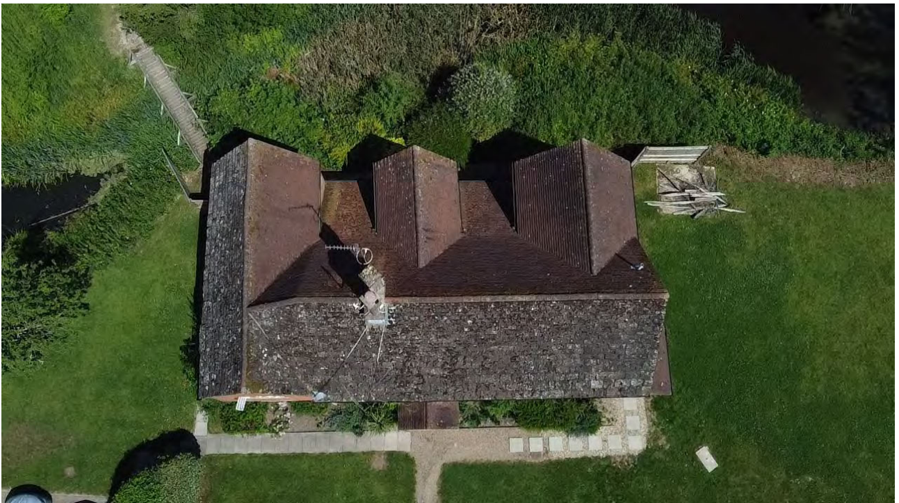
Photograph 2: Aerial view of the Moated House roof (courtesy of L&G)
