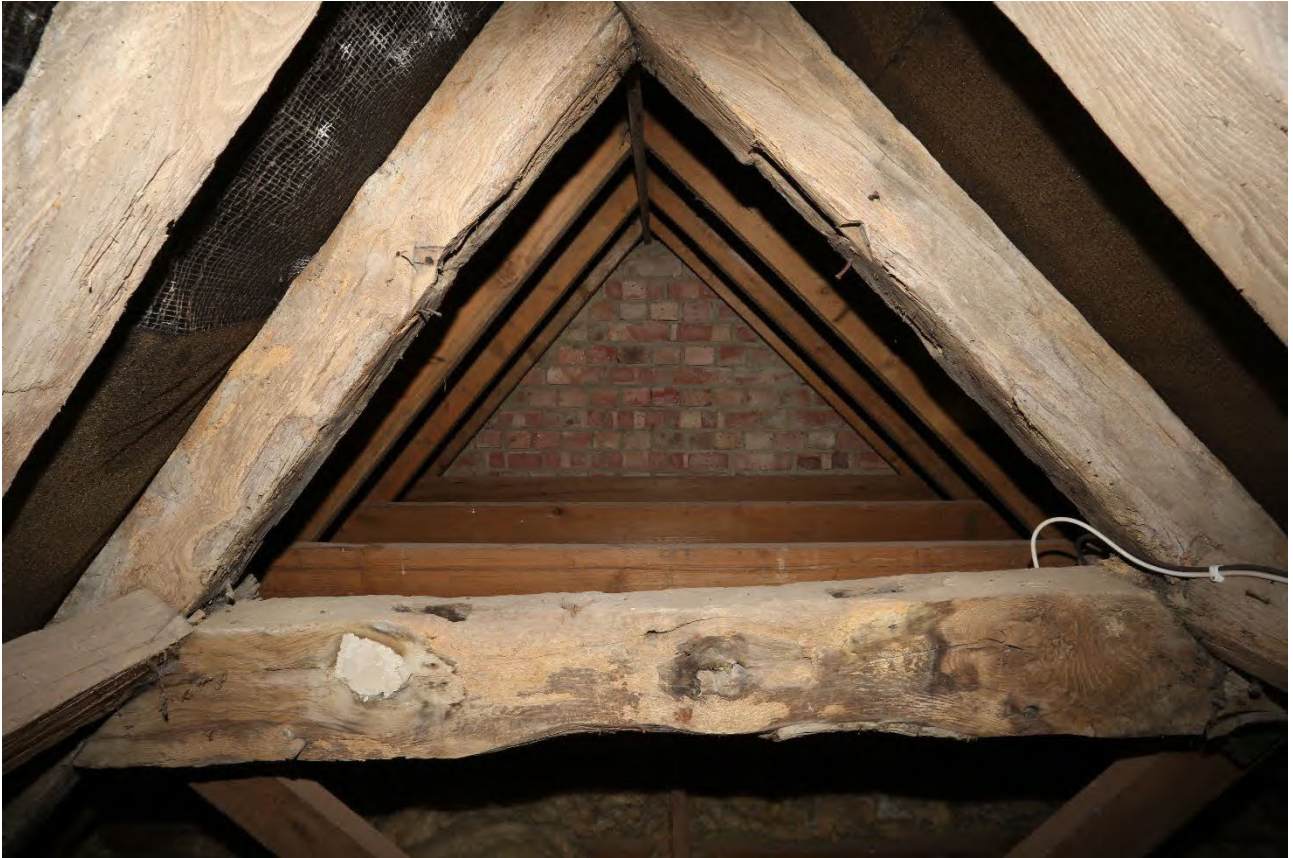
Photograph 1: Surviving historic roof beams within the Moated House (west end bay)
