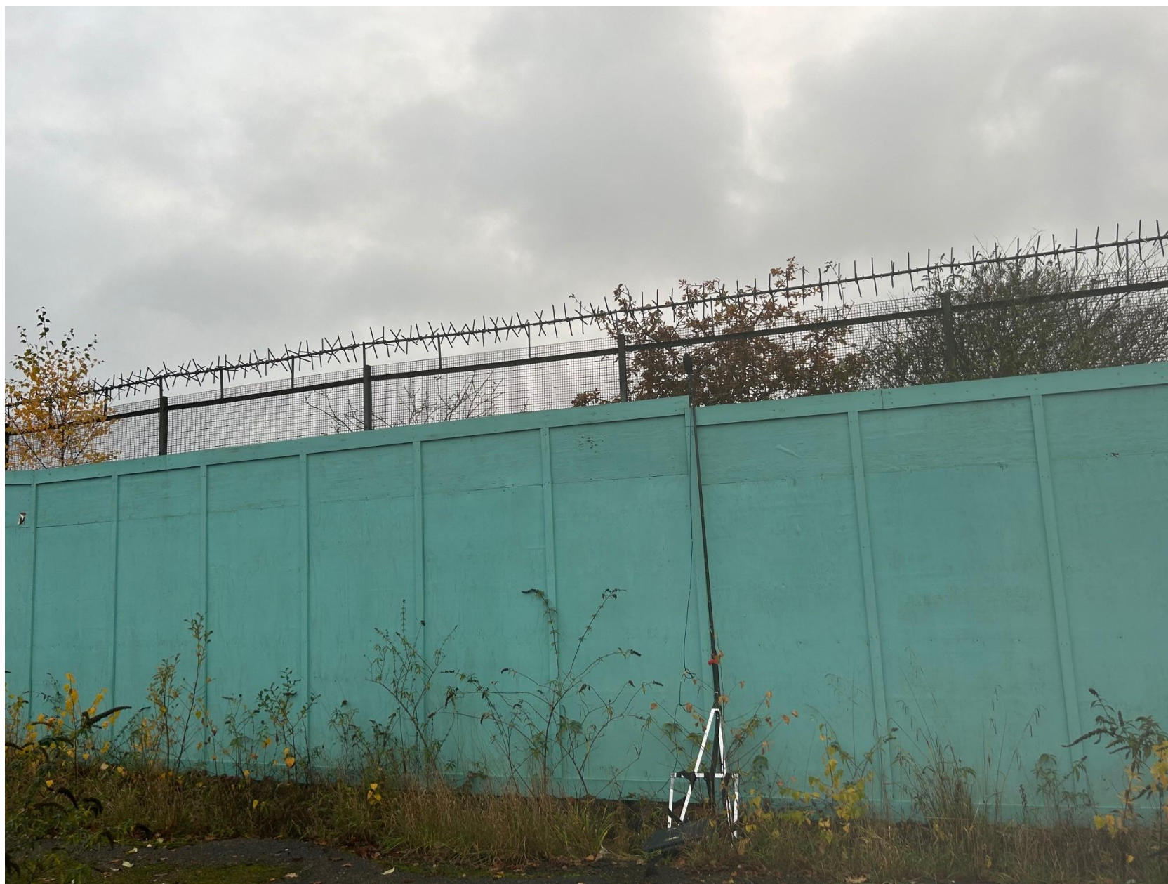
Figure 5 – Photo Showing Measurement Position 4
