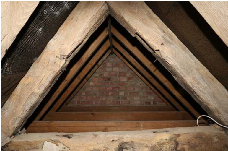
Surviving historic roof beams within the Moated House (west end bay)
