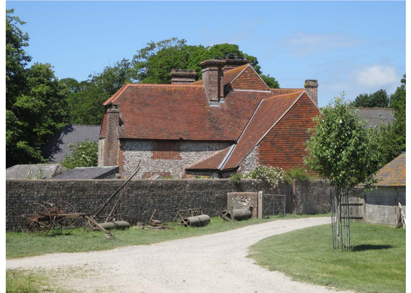
Farm groupings / roofscape variety
