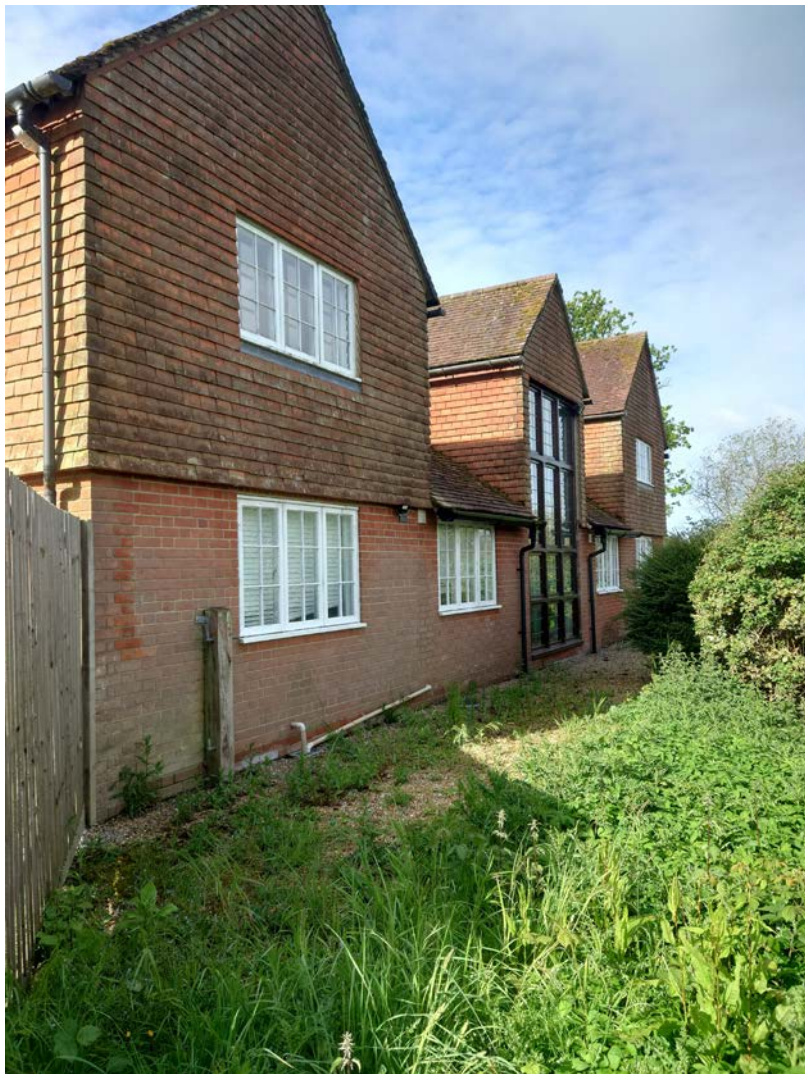
View 2: rear elevation of the farmhouse
