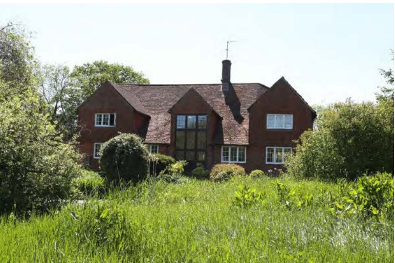
The rear of Moated House viewed from across the moat
