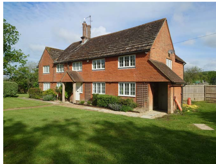
View 4: the front elevation of the farmhouse
