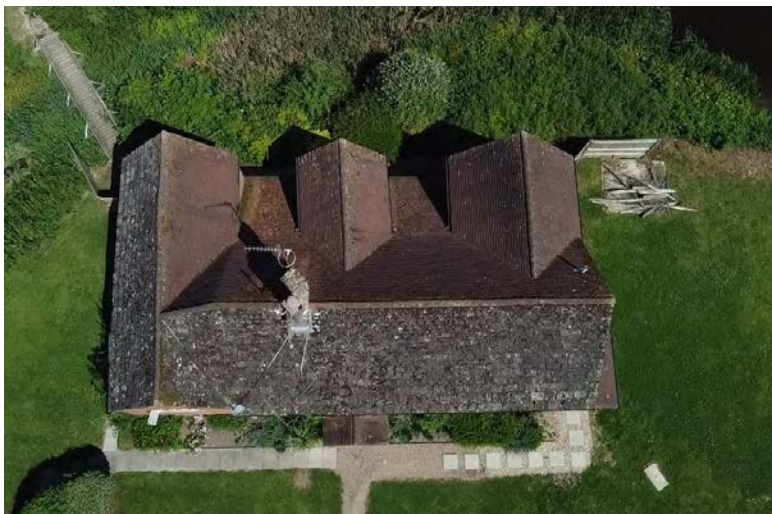
Aerial view of the Moated House roof showing use of original Horsham stone tiles and replacement concrete plain tiles (courtesy of L&G)
