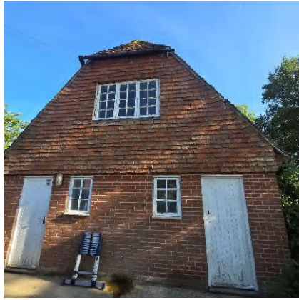
Photograph 7. Garages (MH2) north elevation.
