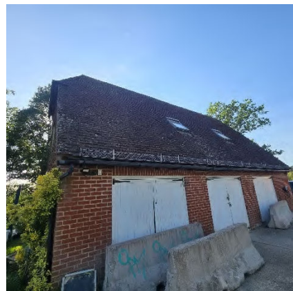
Photograph 6. Garages (MH2), west elevation
