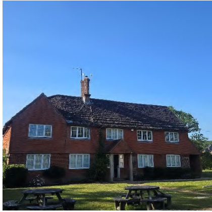
Photograph 1. Farmhouse (MH1) front (south) elevation.
