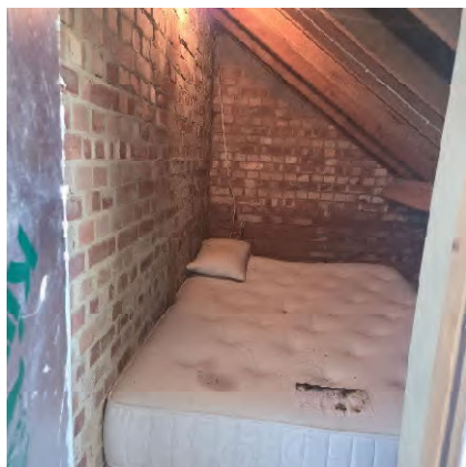
Photograph 5. MH1 roof void 2.
