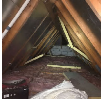
Photograph 8. MH2 internal loft void
