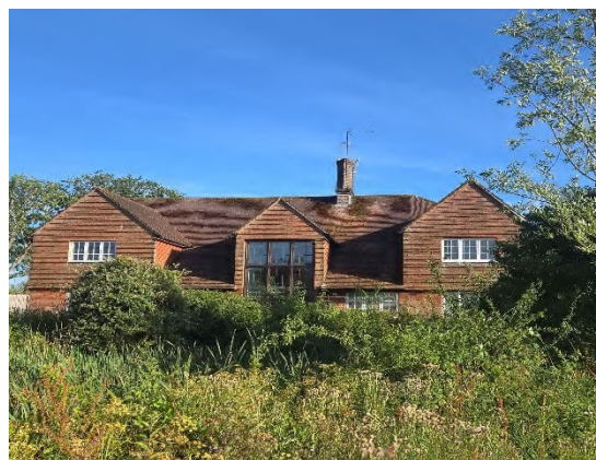
Photograph 2. Building MH1 north elevation taken from north bank of moat with tall ruderal, scrub and bulrush of moat bank tops present in foreground.
