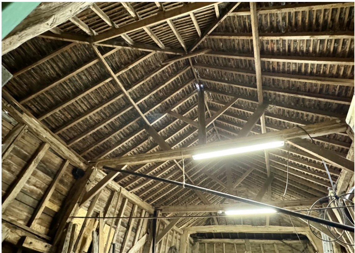
Fig 4: The proposals do not relate to the historic tithe barn. The author of this report has had access to the historic tithe barn and is satisfied that its timber frame structure and historic fabric remains unaltered.
