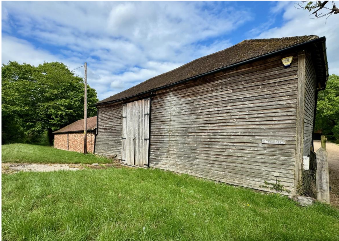
Fig 3: The tithe barn is believed to date from the 18 th Century if not earlier. Its principal elevation faces the highway and it is from here that the significance of the curtilage outbuilding is best appreciated ( see 3.2 ).
