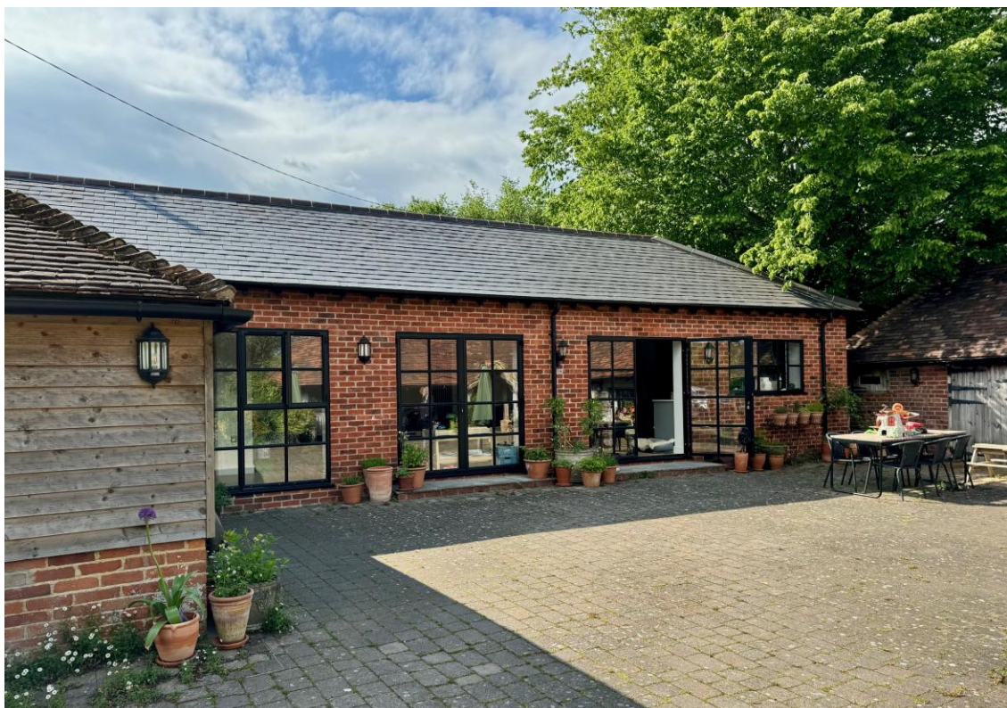
Fig 10: A Victorian single storey extension to the north shown on the tithe map is brick built with a slate roof and the proposal has maintained this later use of materials, repairing and replacing them as necessary.
