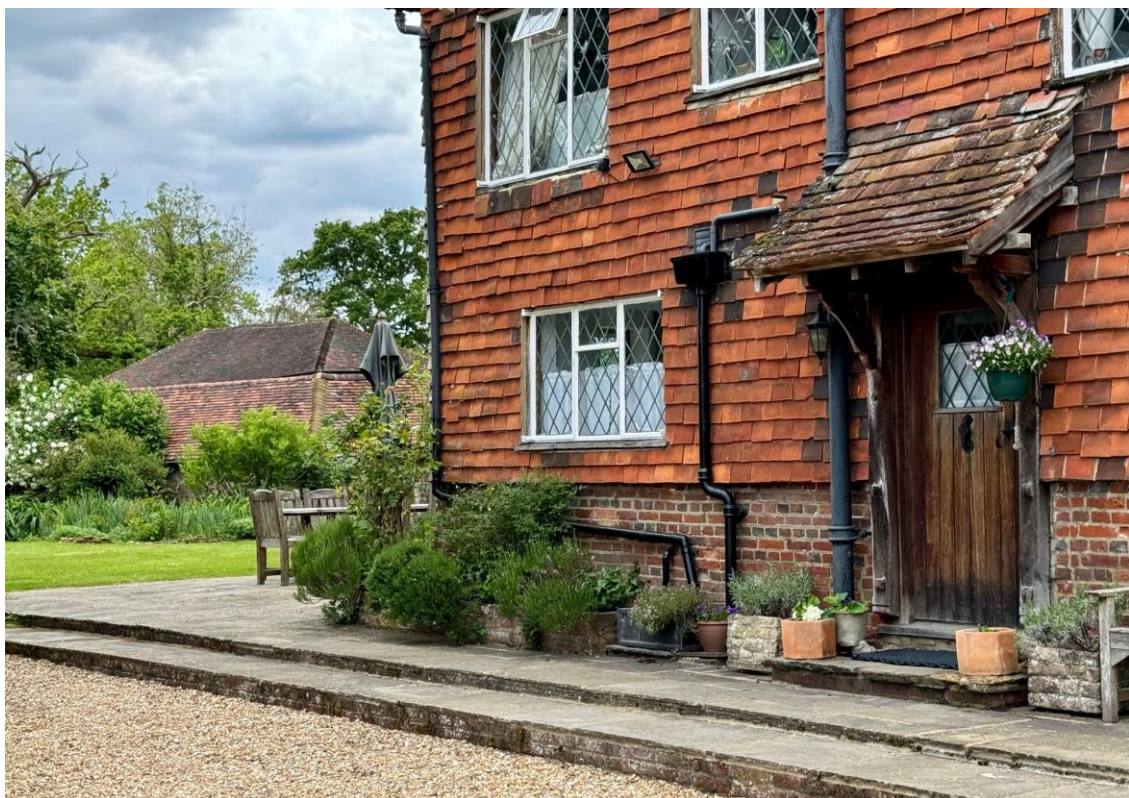
Fig 6: The principal elevation of the former farmhouse faces east overlooking the driveway, as seen here. Due to proximity, the dwelling maintains a close association with its range of curtilage outbuildings.
