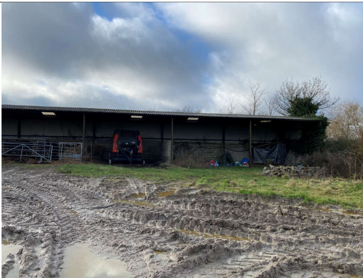
Photo 3: View South of Southern Barn
