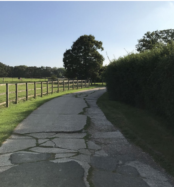
View from the north towards the site entrance and the mature oak tree.
