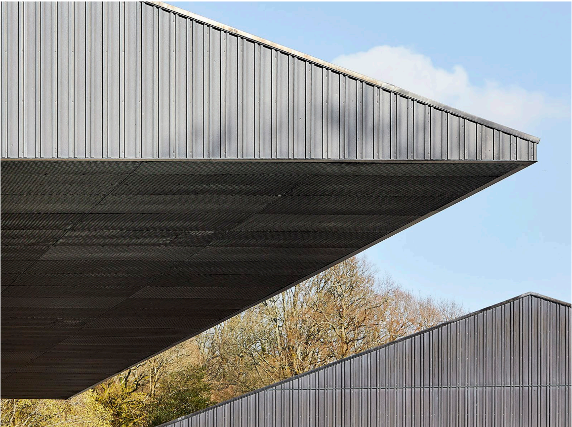
Wall cladding and overhanging eaves in fully oxidised copper cladding
