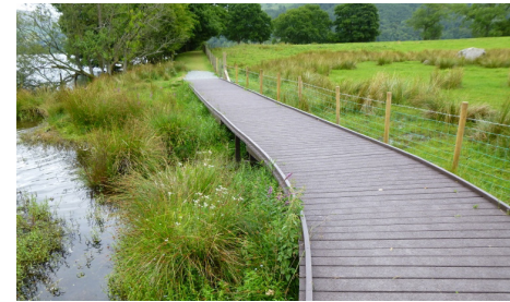
Pedestrian bridge crossing the stream
