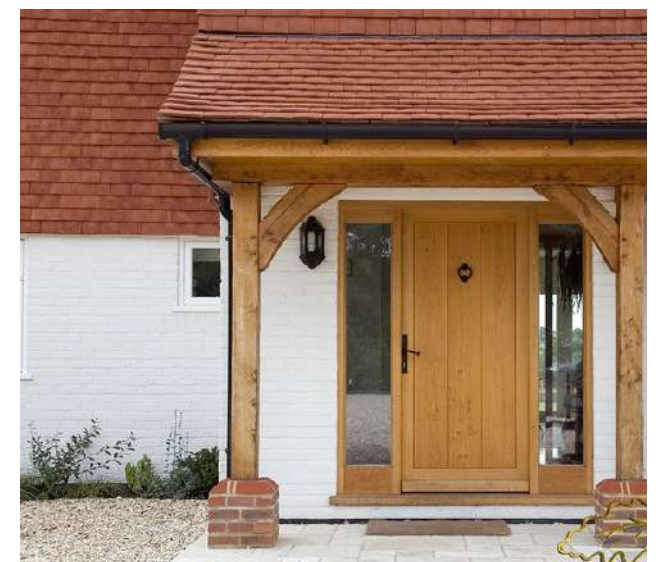
9. Timber Porch with Brick Plinth
