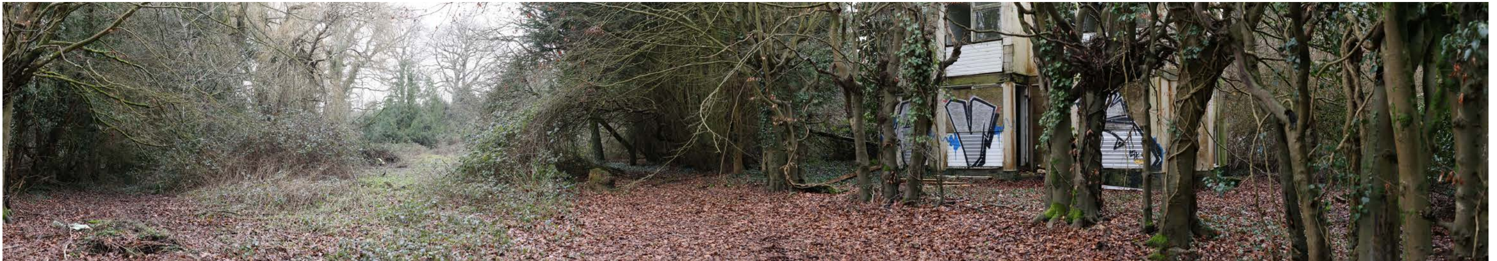
Site Photograph B. Poor state of repair of built form on Site, with beech tree line about the south western boundary of the Site.
