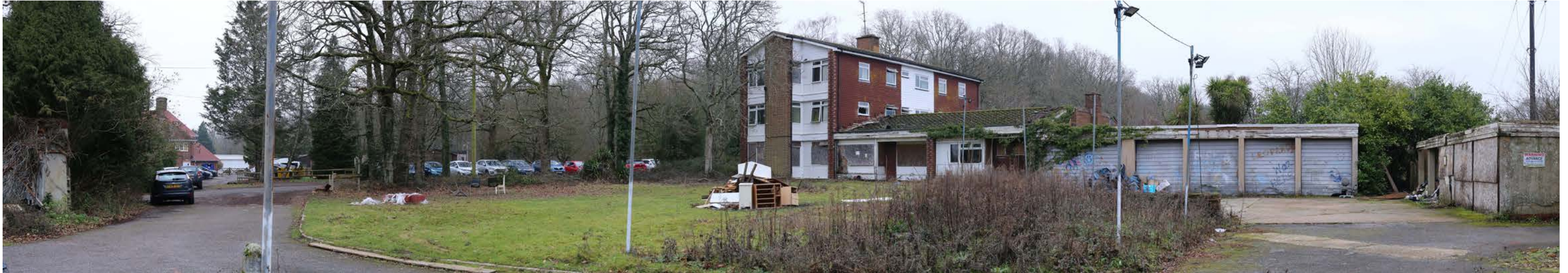
Site Photograph A. North easterly perspective from Woodland Close within the Site.
