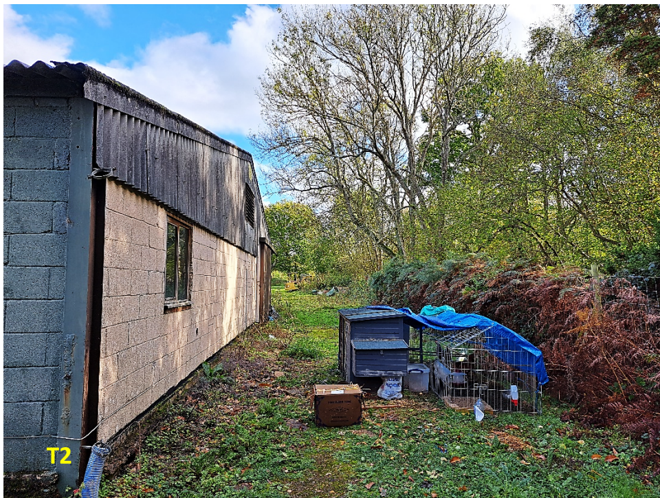
Photo 2 (above): The rear of the existing barn
