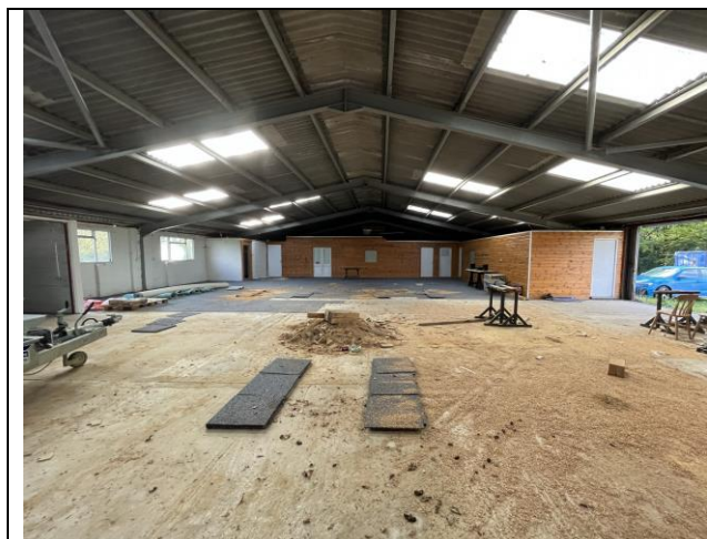
Photograph 7: The farm building internal with void above the offices.
