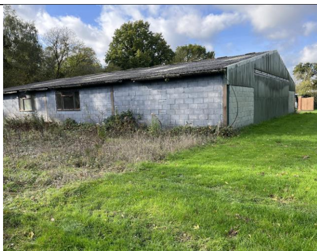
Photograph 6: The north and east elevations of the farm building.
