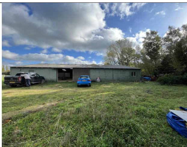
Photograph 5: The west elevation of the farm building.
