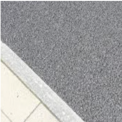
Tarmac to adoptable pavements and the main road.
