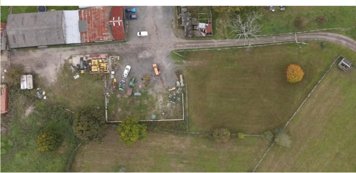
Overview of site
