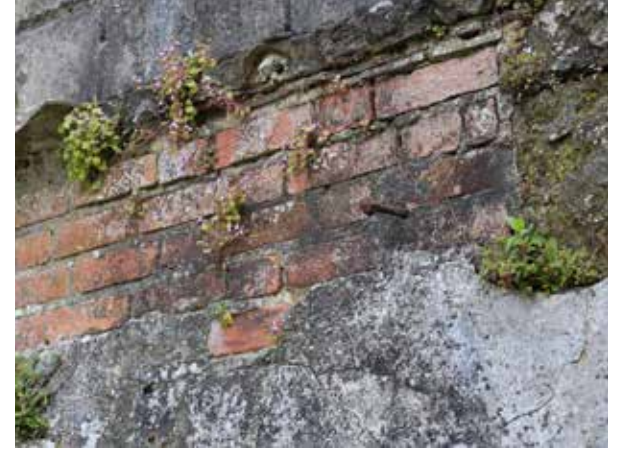
Photograph of existing wall of the barn
