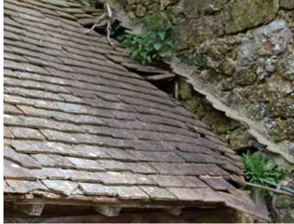
Photographs of existing roof of the barn
