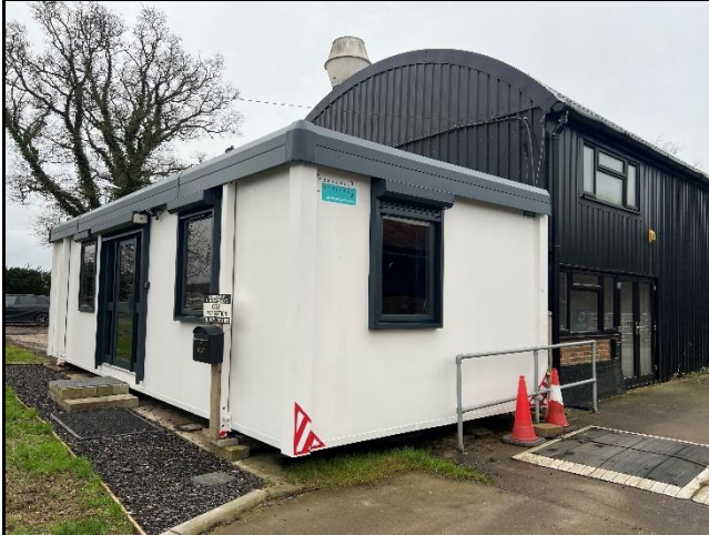
Portakabin to the north-east of Building '4'.
