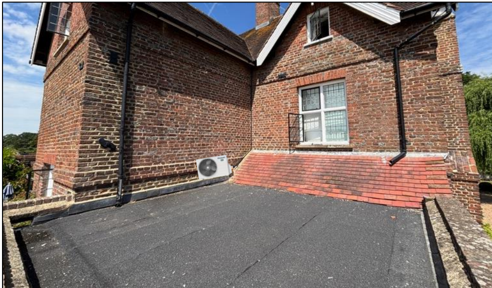
Condenser design location – before spray paint
