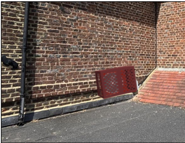
Flat Roof east side (above reception room)
