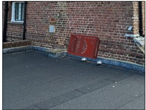
Flat Roof west side (above kitchen)
