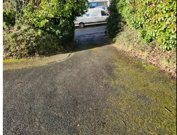
Photograph 8 – Tarmac access drive.
