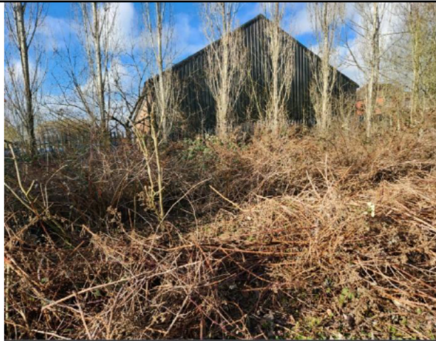
Photograph 5 – Western border bramble scrub.
