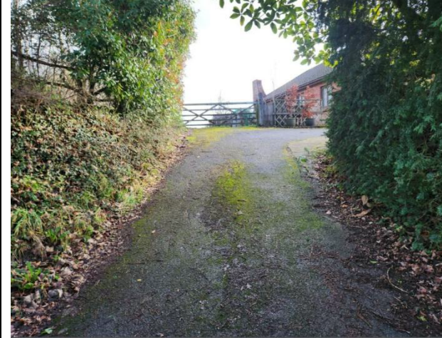
Photograph 7 – Tarmac access drive.
