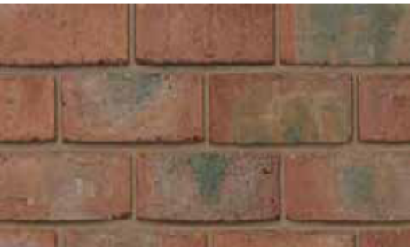
Red Brick Detailing
