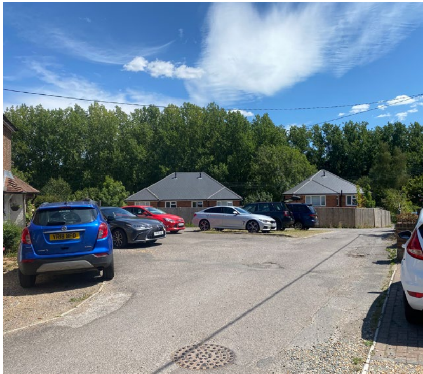
Montpelier Gardens Parking Areas
