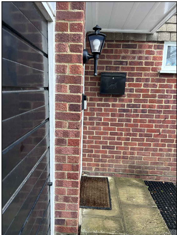
3 - Side View (Entrance)
