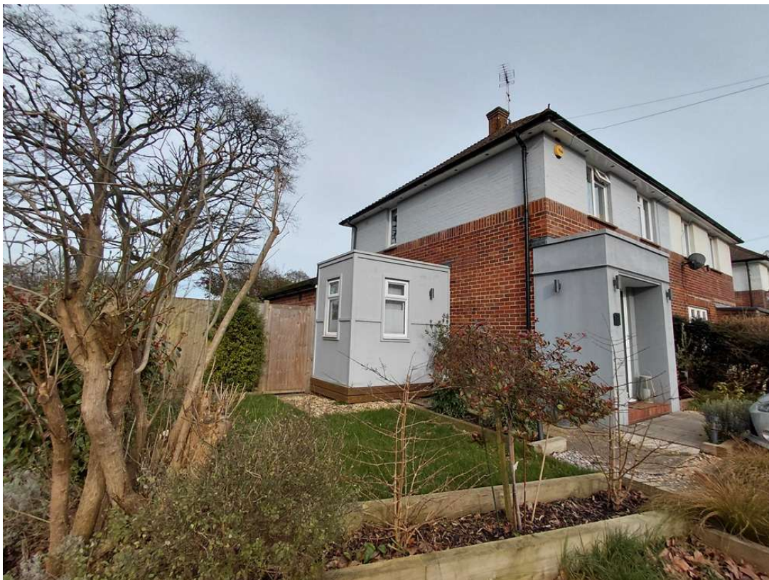
Front-side of Subject Site- No. 25 - Above
