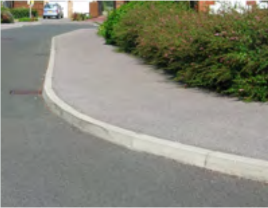
Tarmac to primary road and public pavements
