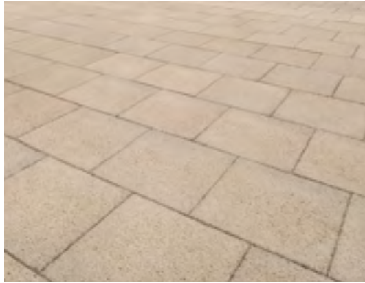
Paving slab to front garden path
