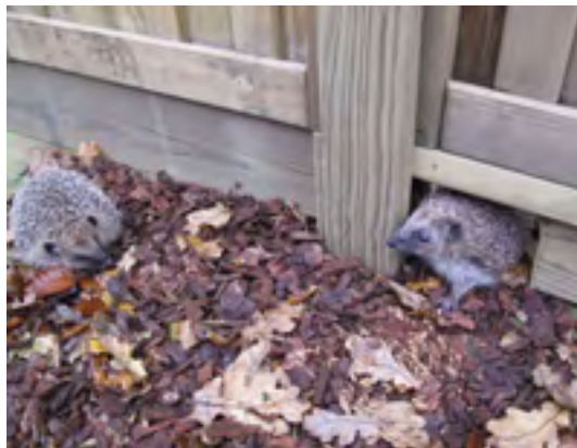
Closed board fence with hedgehog gravel boards
