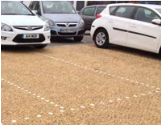
Stabilised gravel to allotment car park
